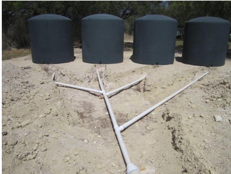
COLLECTION TANKS (3K GALLON) CONNECTED TO PLENUM
