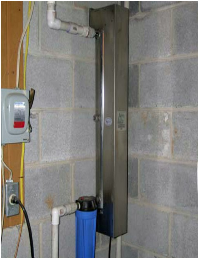
Figure 2. A typical UV light installation with a small canister sediment filter (bottom) ahead of the UV light unit.
