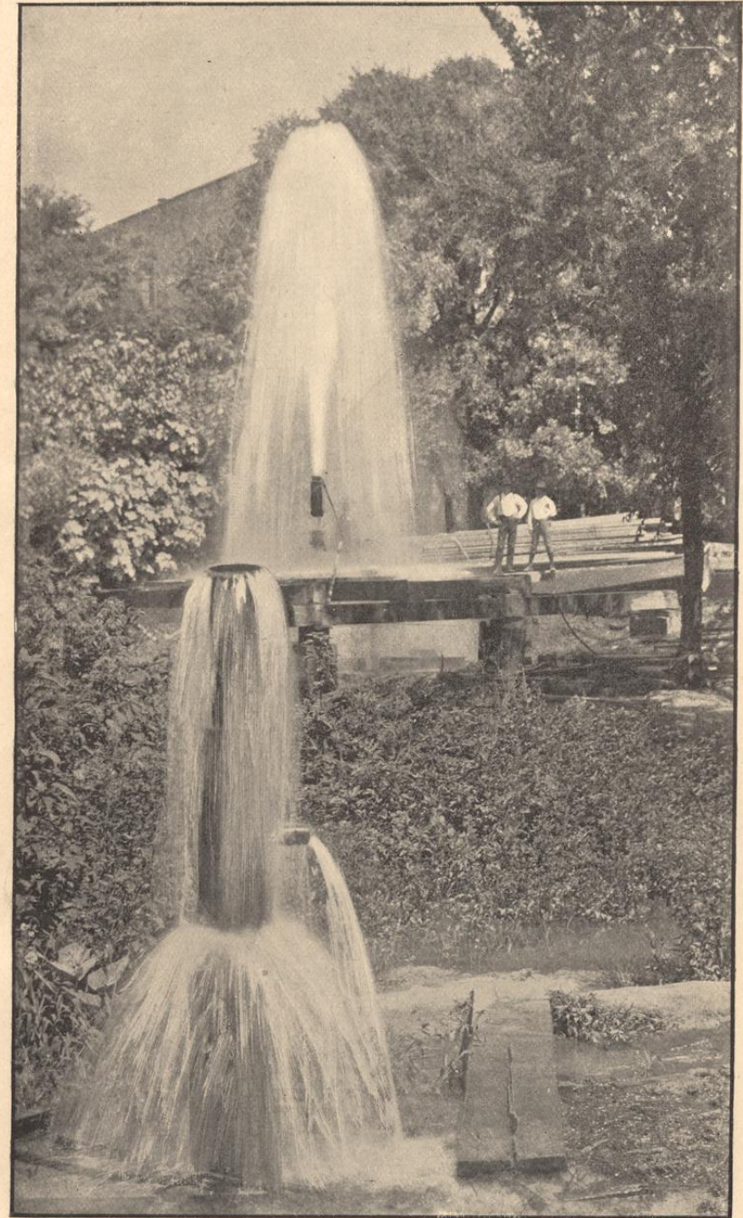
ARTESIAN WELLS AT CITY WATERWORKS, SAN ANTONIO.
